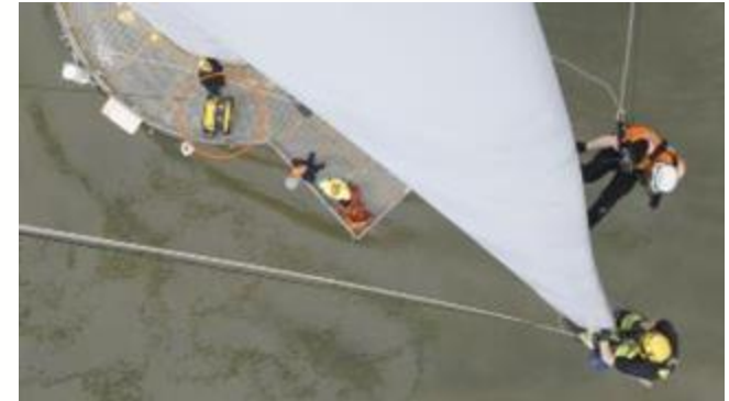
Technicians inspect blade controlling position with Limpet
