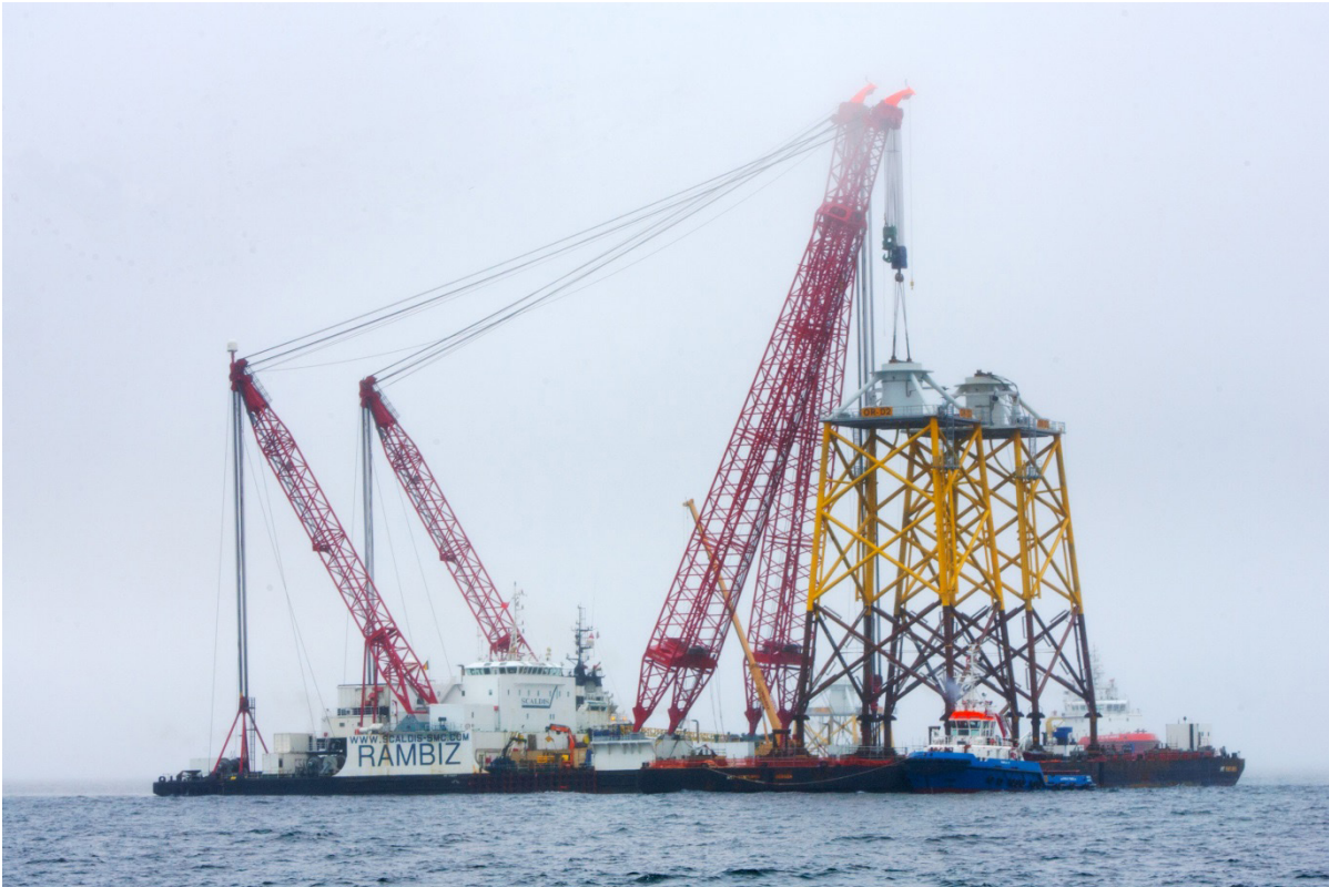
Figure 3: Jacket foundations being installed at Ormonde
