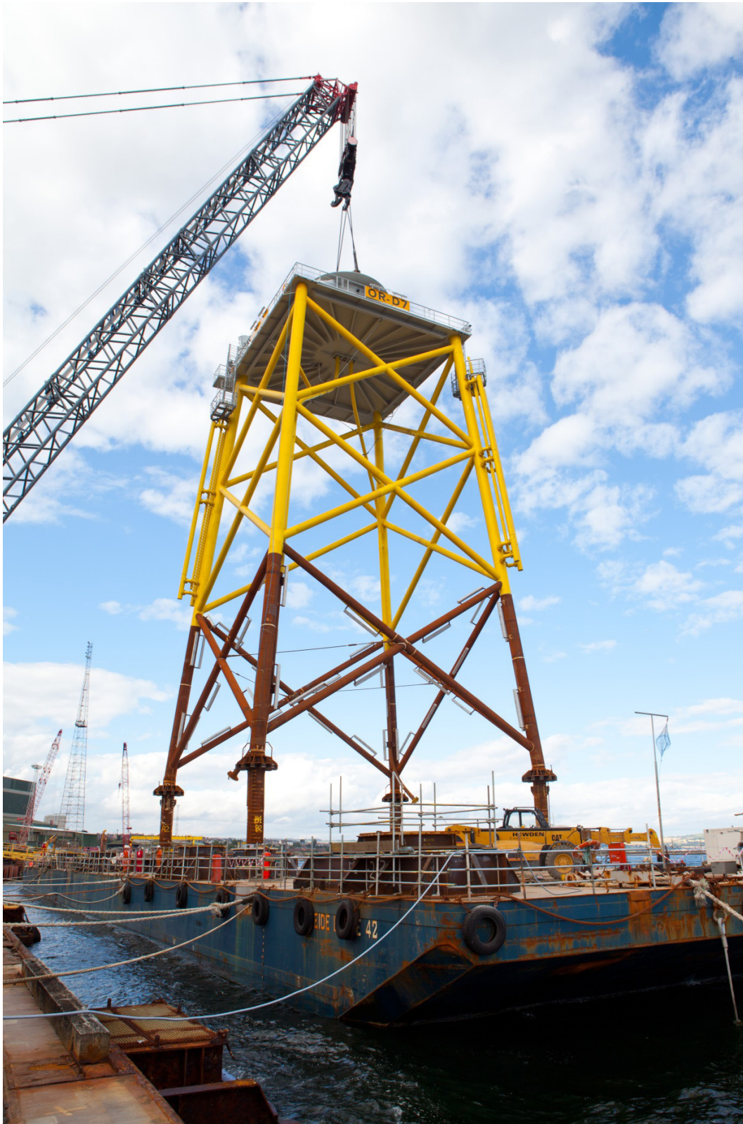
Figure 2: The OWEC Quattropod® jacket foundation installed at Ormonde
