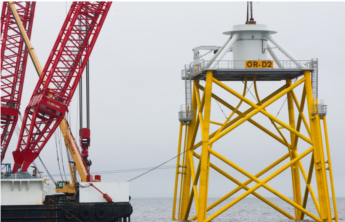
Figure 4: The Ormonde jacket foundation installed at the site
