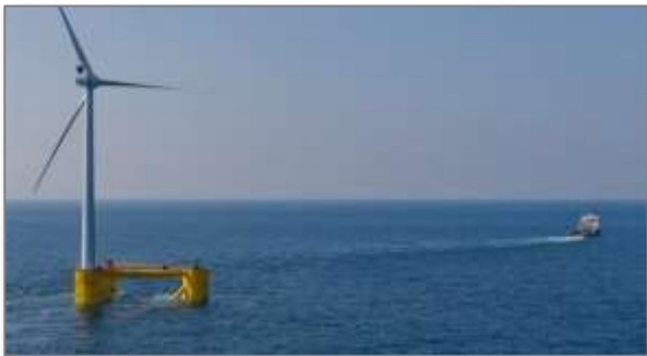
Figure 3 WindFloat Installation in Portugal (Source: http://www.marineitech.com/ )
