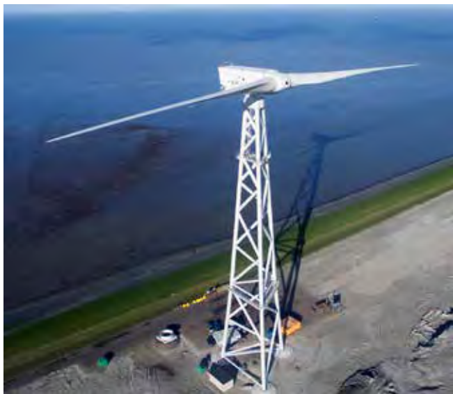
Figure 2. The 2B Energy 140-m, 6-MW downwind wind turbine in Eemshaven
