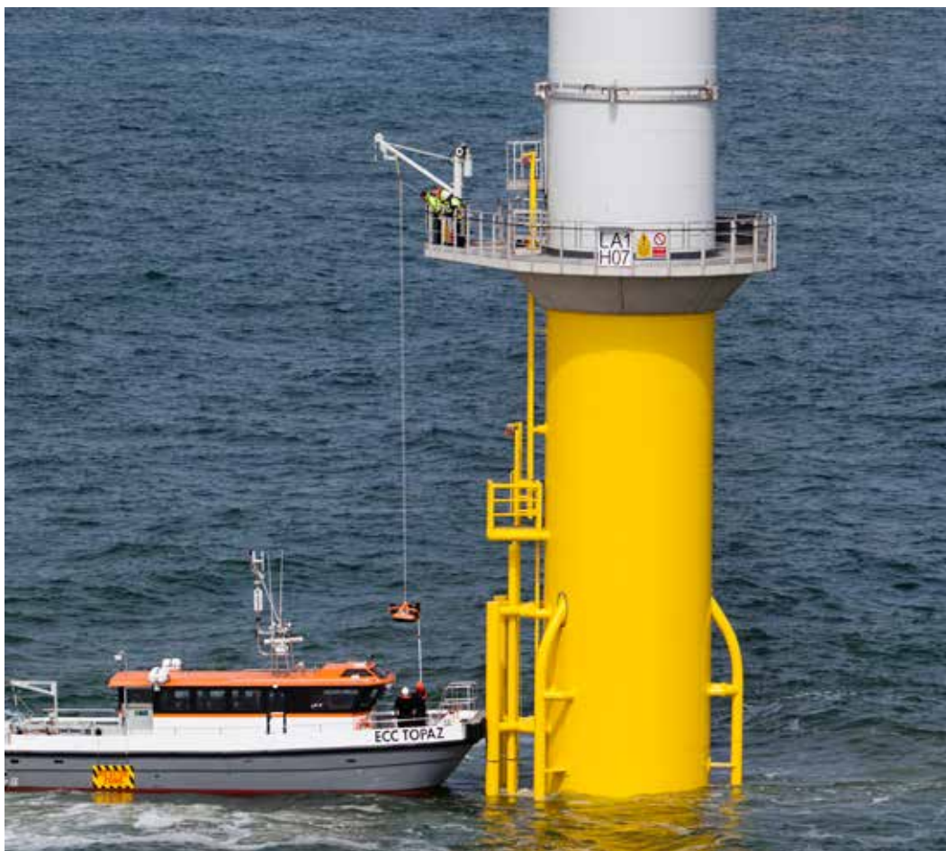
Figure 4: Technicians transfer to a turbine at London Array. Credit: www.siemens.com/press
