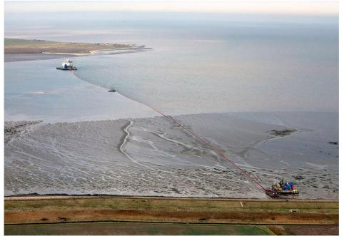
Figure 2: Illustration of shore pull during cable lay. Image courtesy of VBMS.
