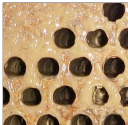
Figure 10c. A Slime Layer/Biofilm on Heat Exchanger Tubes in a Commercial Ship.
