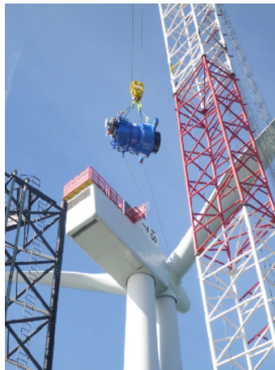
Figure 3: Change-out of a Winergy gearbox at Sheringham Shoal in Q1 2015
