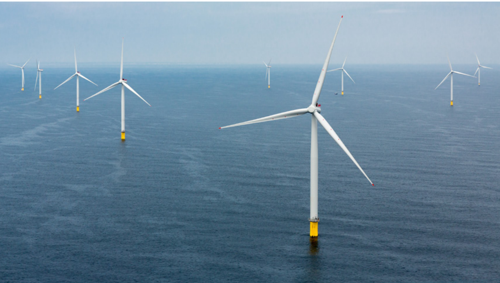
Below: Westermost Rough Offshore Wind Farm (Image: Siemens)
