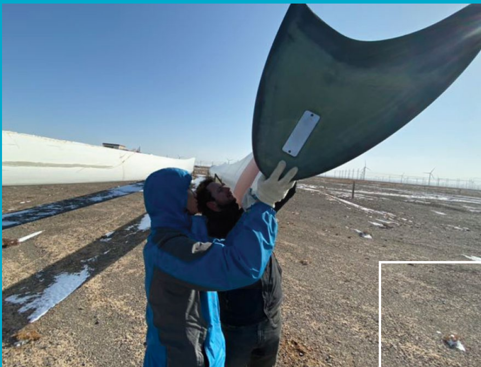
Anakata's 'winglets' technology being fitted to a wind turbine blade.
