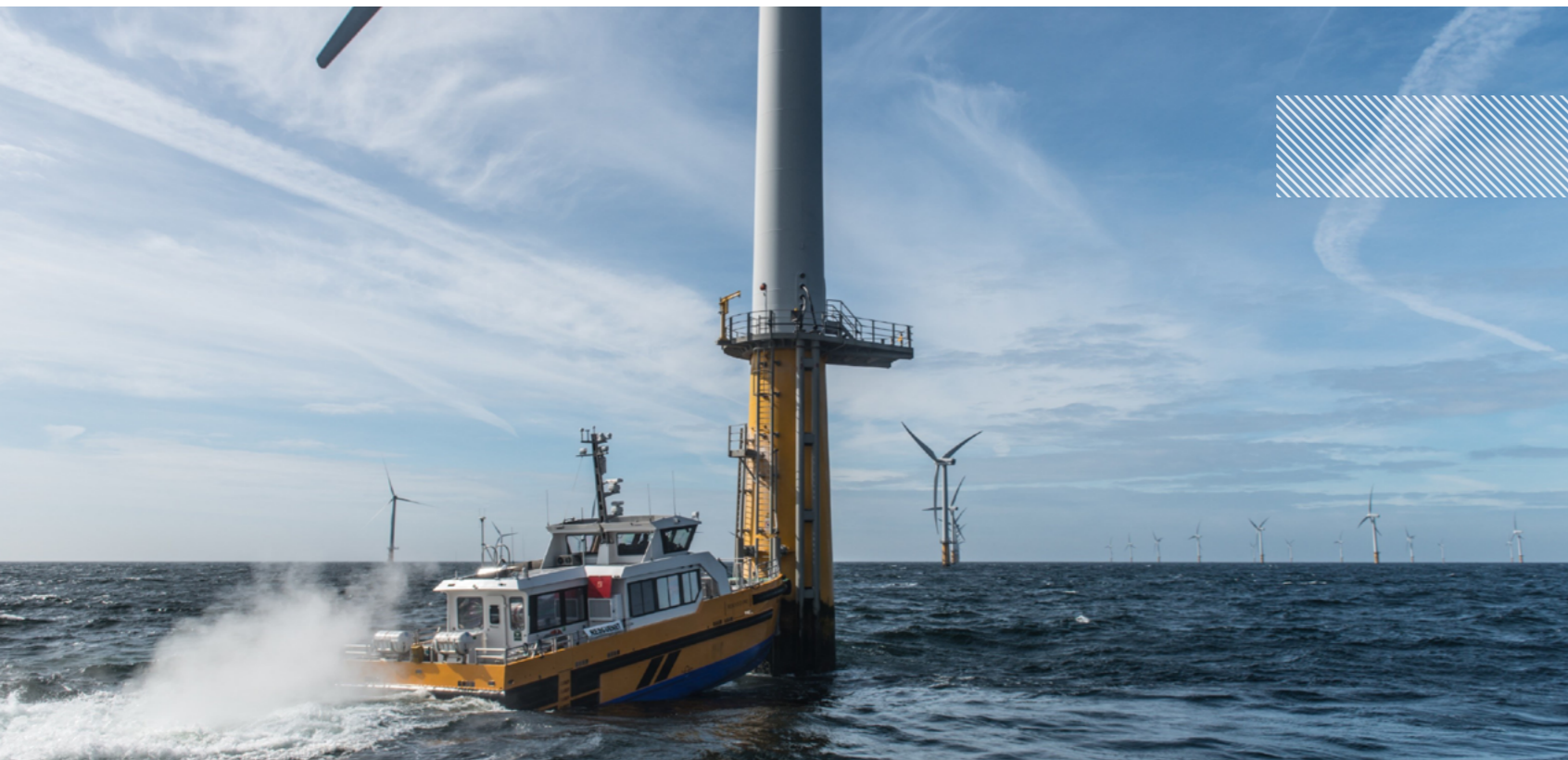
A crew transfer vessel approaching an offshore wind turbine
