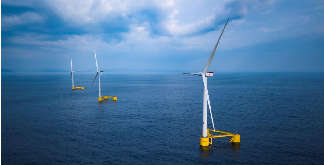
WindFloat Atlantic final hookup at Viana do Castelo, Northern Portugal (Credit: Principle Power)
