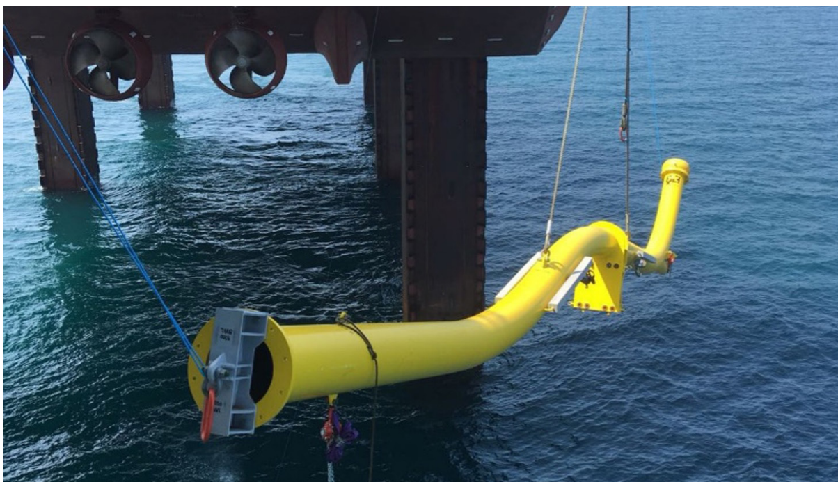
Figure 12: Cable J-tube (Courtesy: Optimus Aberdeen) 13
