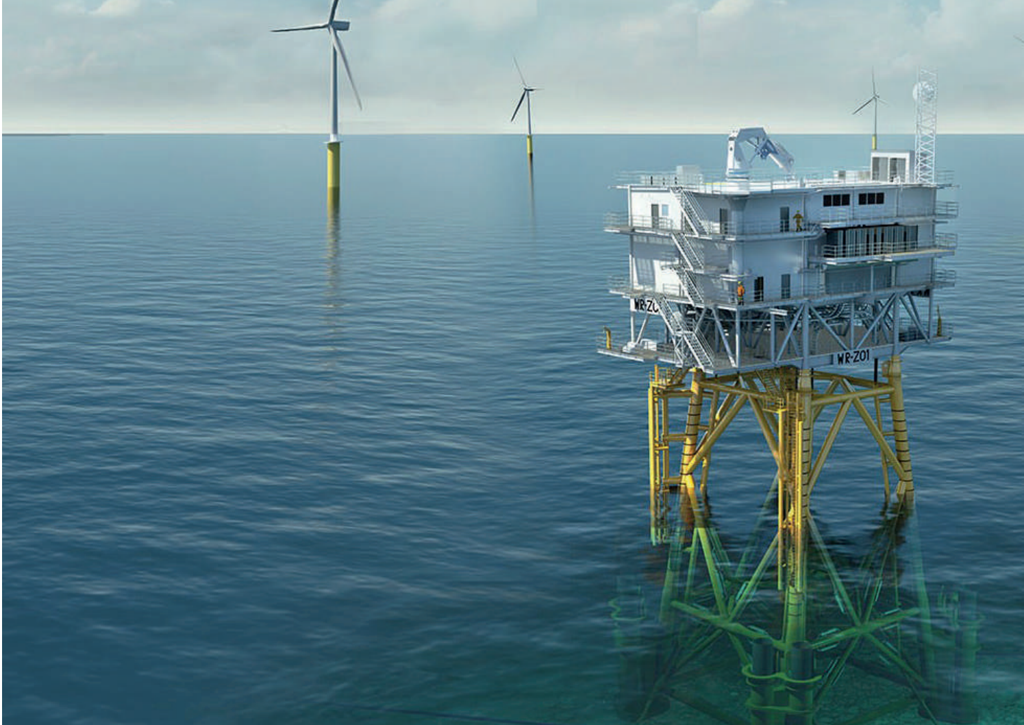
Figure 26. Offshore substation and wind turbine. (Source: Ramboll)
