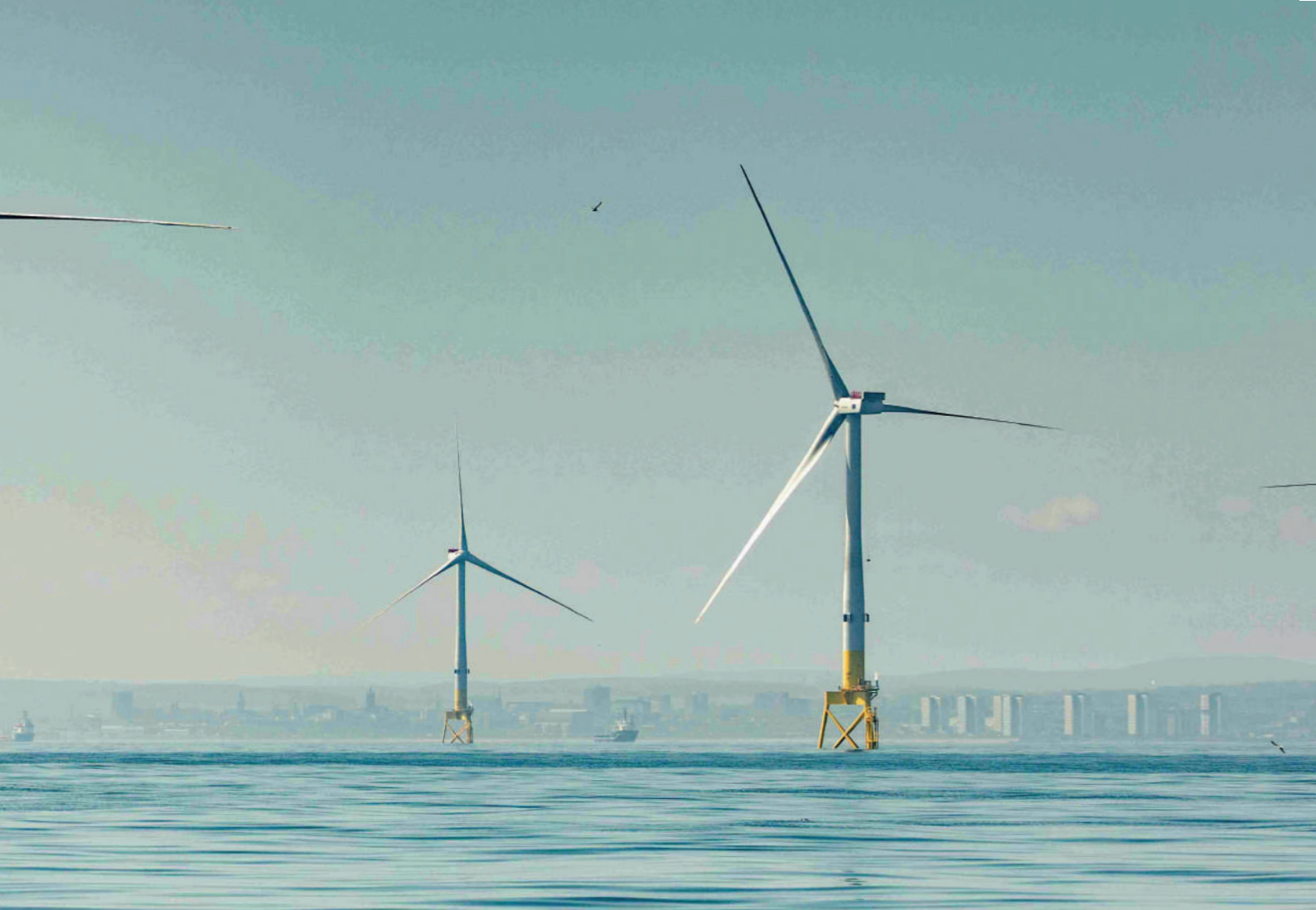
Figure 12. European Offshore Wind Deployment Centre at Aberdeen Bay Windfarm, UK. (Source: Vattenfall)
