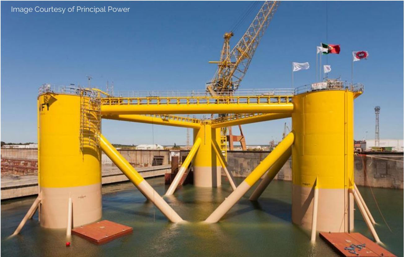
Figure 1 - Onshore assembly... Floating turbines, like this semi-submerged model, can be assembled in harbour or near shore and towed into position
