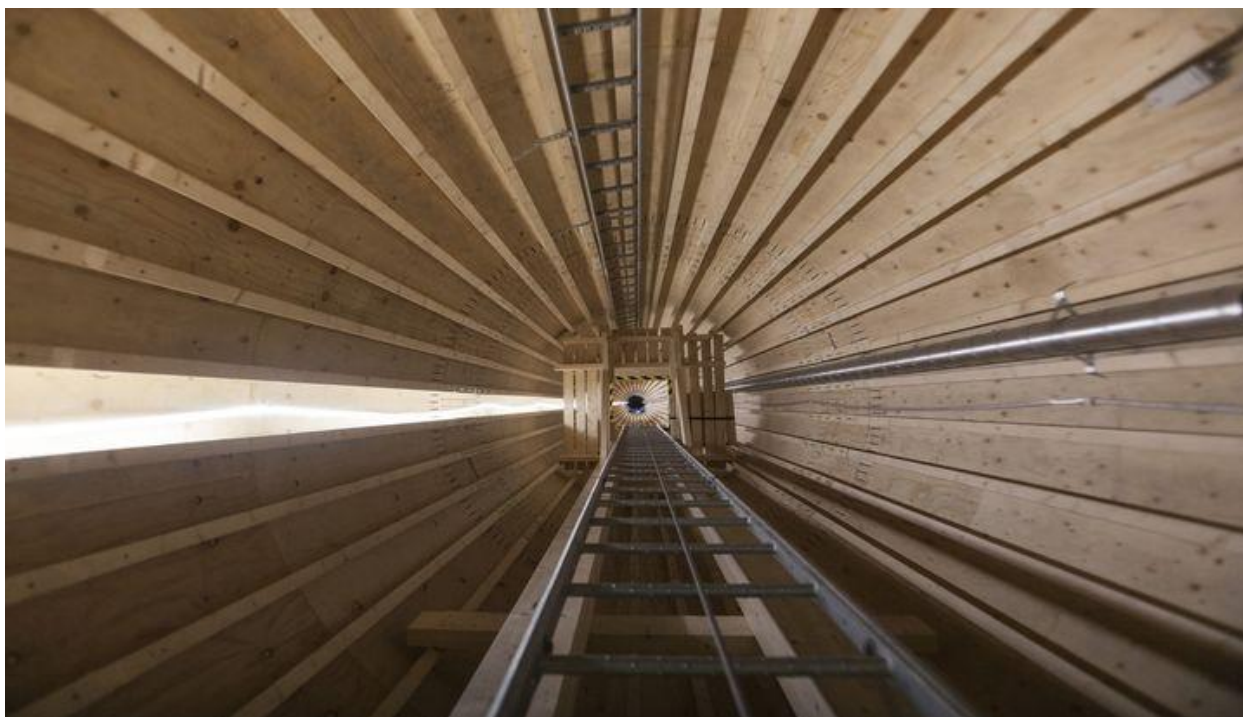
Figure 8: The inside of a Modvion wooden wind turbine under construction. Farmer, M. (2021, May 10). Reach for the sky: A tale of wood and wind. Power Technology. https://www.power-technology.com/features/reach-for-the-sky-a-tale-of-wood-and-wind/
