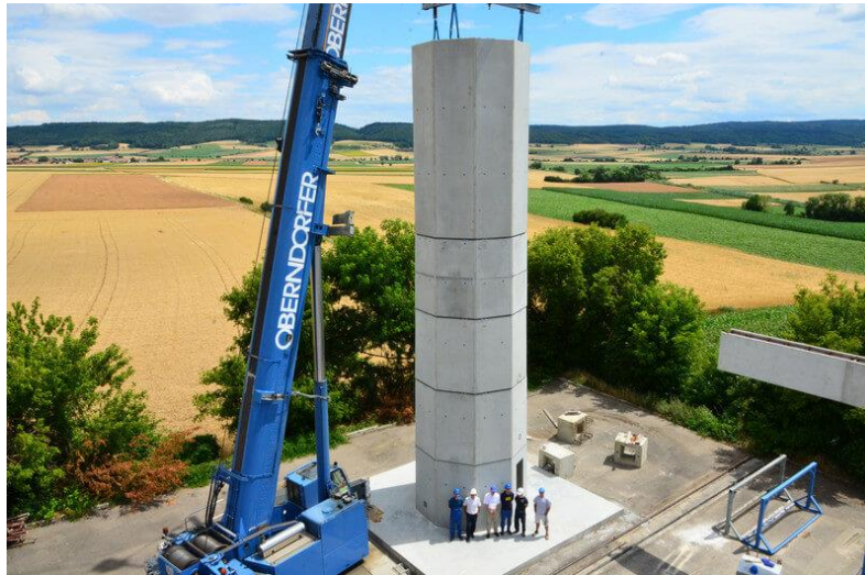
Figure 17: An onshore segmented concrete tower under construction. [16]
