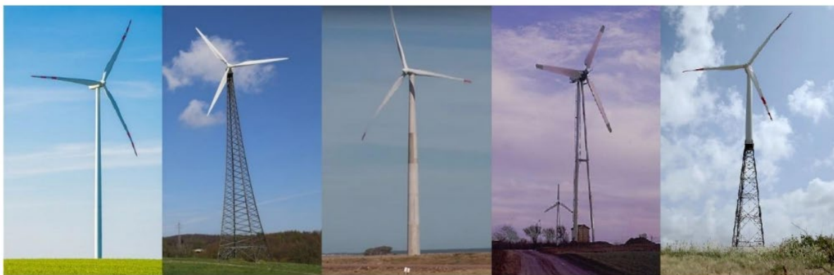
Figure 2: Types of wind turbine towers [5]
