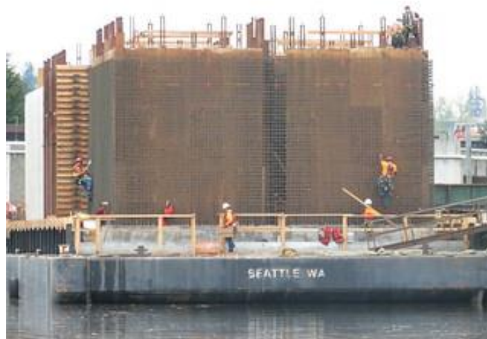
Figure 10: Gravity Anchor Rebar Structure [17]
