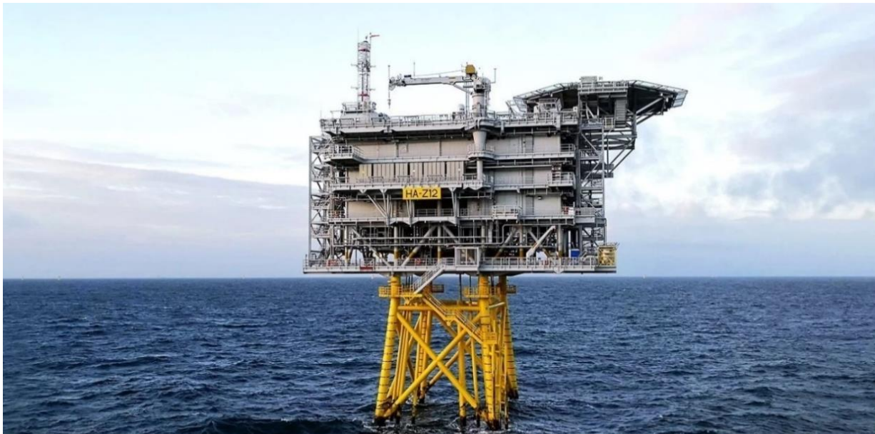
Figure 3: Critical components for the representation of utility-scale offshore wind farms in jacket design [5].
